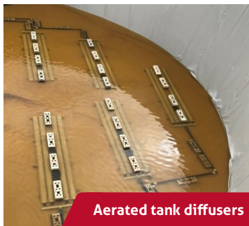
Existing aeration tank and connection to mobile CTP environment units (Biomobil® - Tank)
